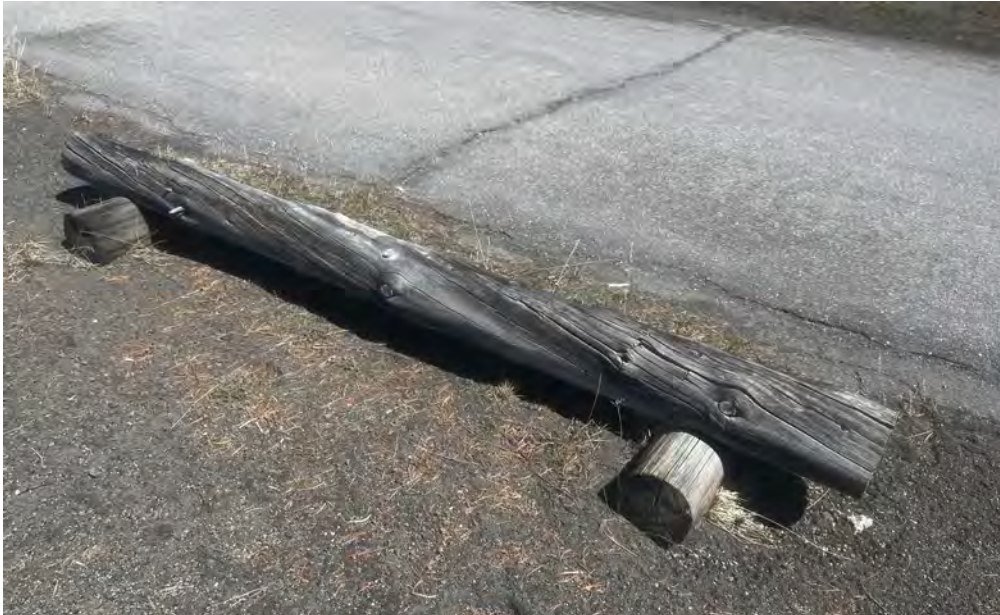
Log barrier to delineate shared path
